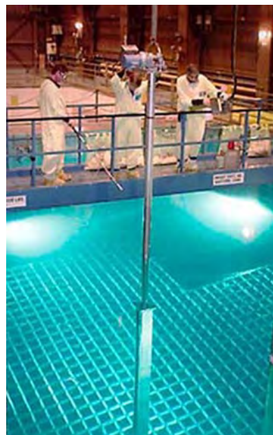
Figure 14.32 Radioactive spent-fuel pool at a nuclear power plant. Spent fuel stays hot for a long time. (credit: U.S. Department of Energy)
