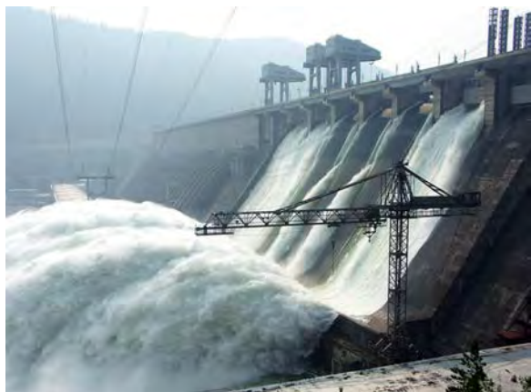
Figure 7.38 Hydroelectric facility (credit: Denis Belevich, Wikimedia Commons)
